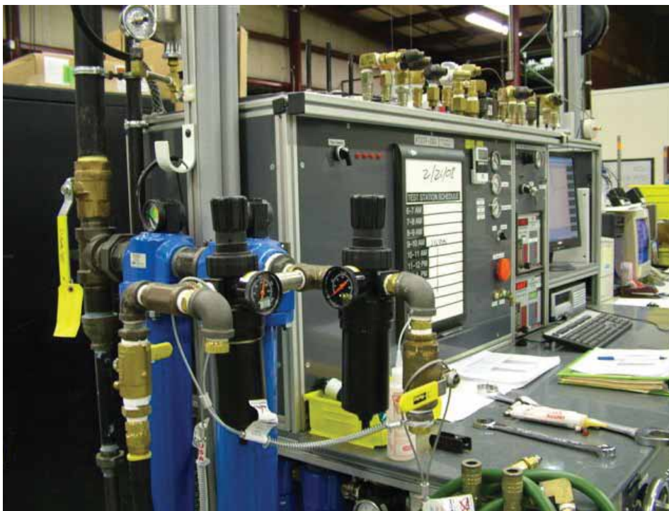
Critical test station serviced with Balston Filter Regulators and Large Prefilters
