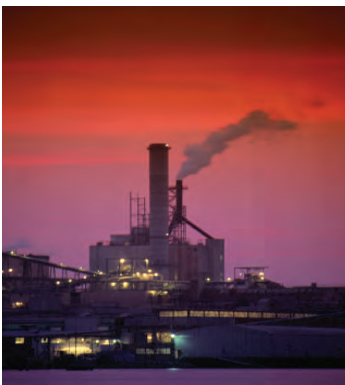
Sample and Instrumentation Filtration
